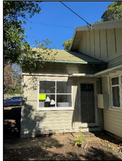
Figure 129. External view to the south-eastern corner of dwelling showing the side of the enclosed verandah. Note non original entry door and fixed timber window.
